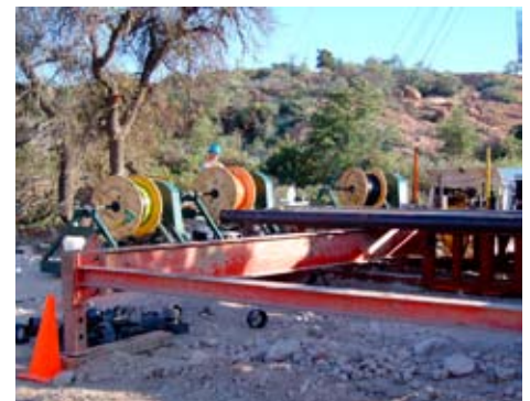
Fiber optic cables before downhole installation at a copper mine.
