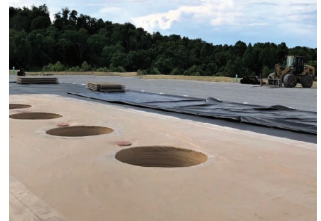
GROUNDGUARD Slip Resistant 16 oz non-woven geotextile backing bonded to 40 mil HDPE
