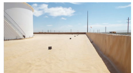
5' height containment lined utilizing tan GROUNDGUARD on the walls and floor.
